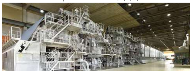
Hood air & Ventilation Balance Controlling system at Paper Machines no. 17, 5, 7, 8, 9
